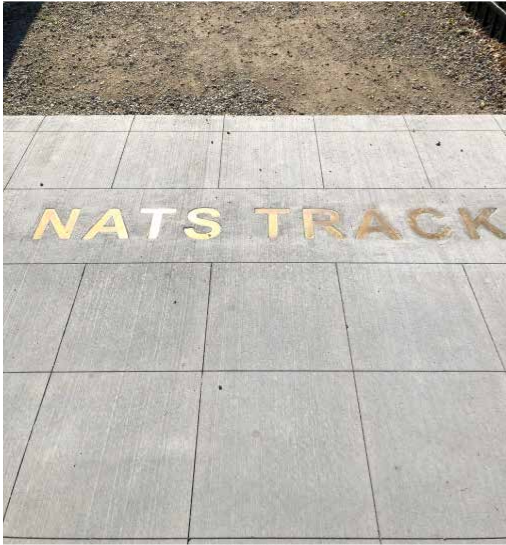
Laser cut text inlaid with insitu paving, saw-paving giving appearance of modular pavers
