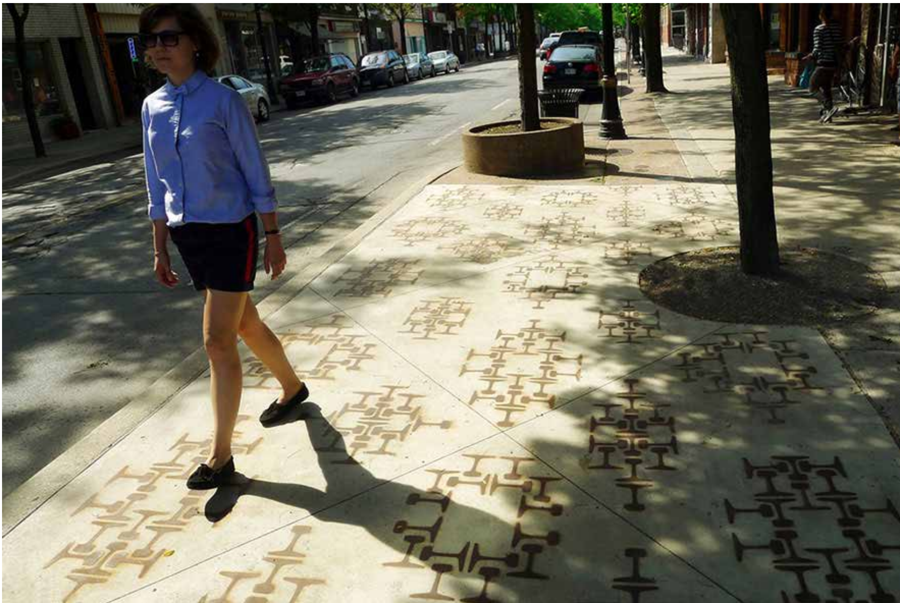
Design narrative: laser cut sections of train rail tracks inlaid with insitu paving
