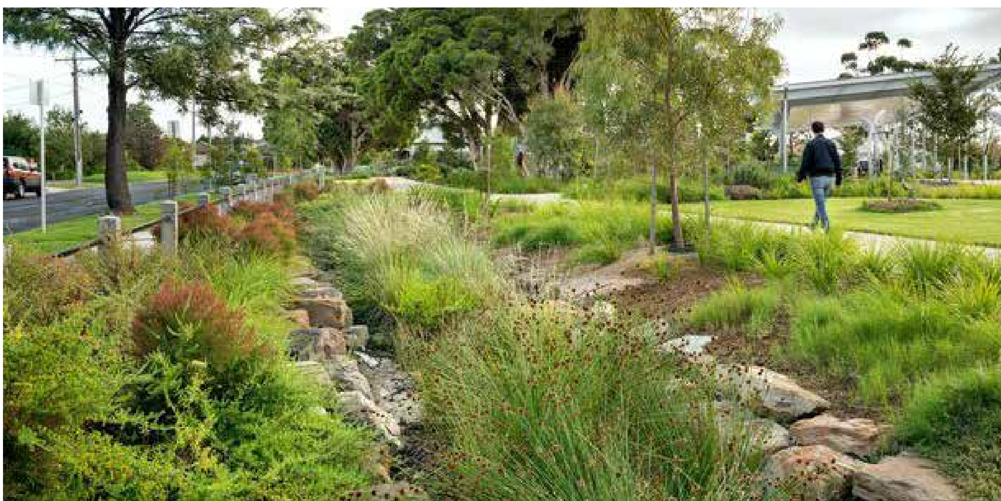
Planted swale / storm-water filtration
