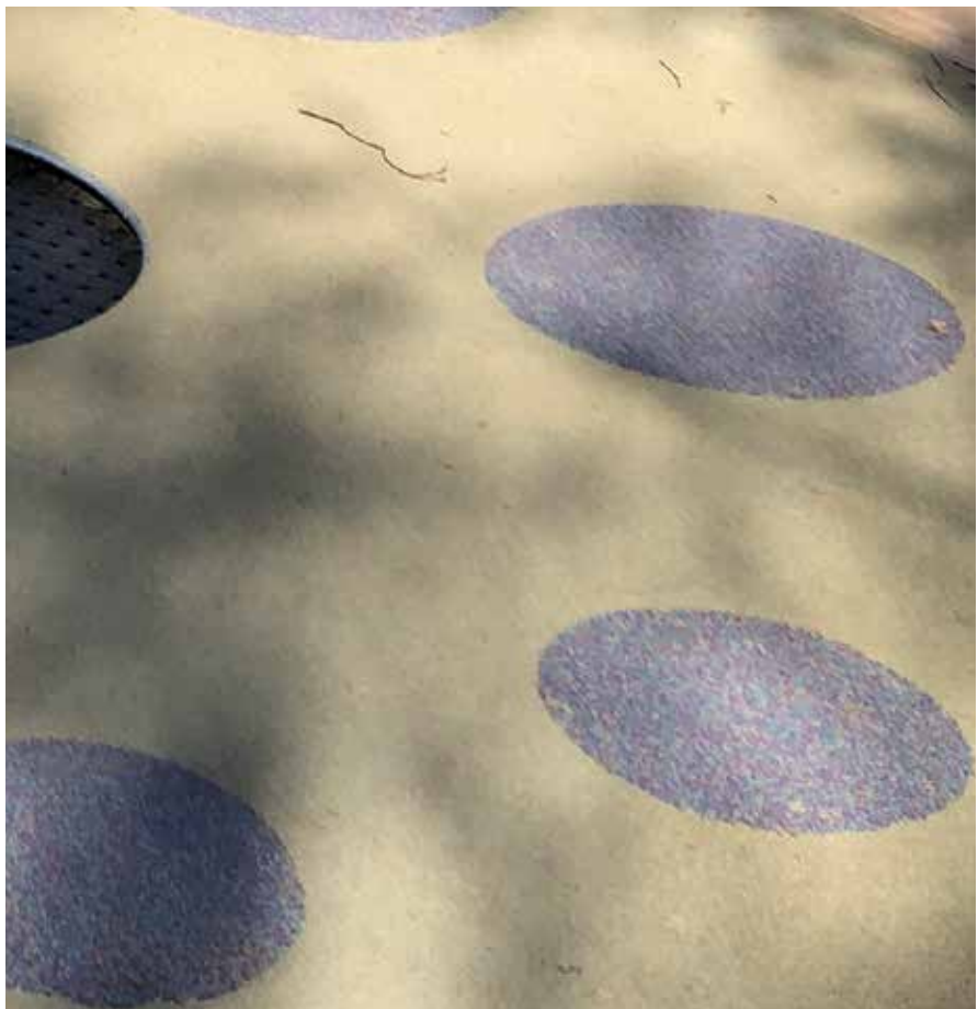
Impact layer rubber surface to play equipment allowing accessible surface
