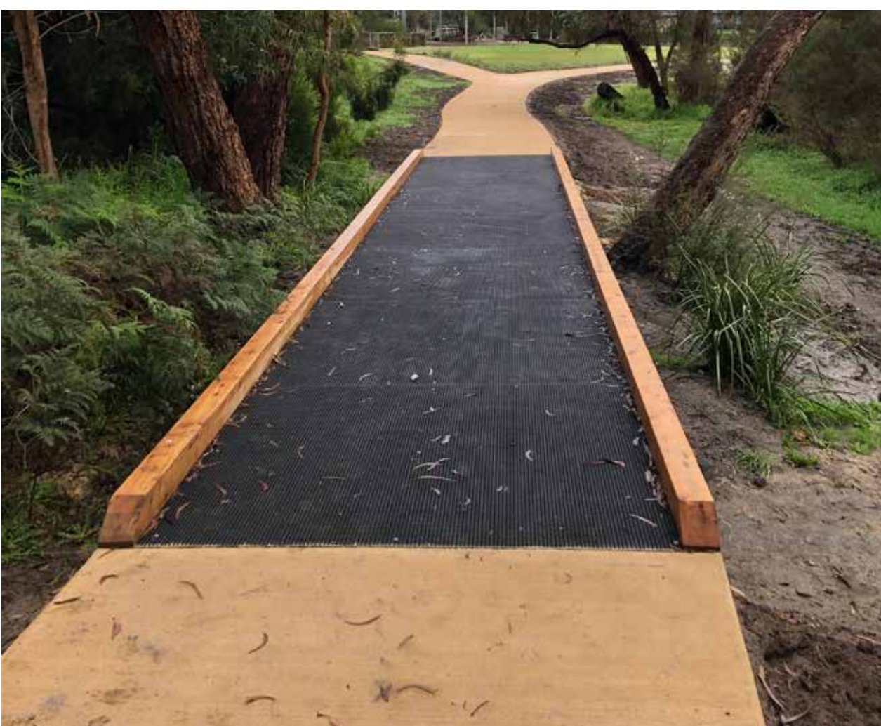
Small pedestrian bridge (FRP mesh) with timber kick-rails
