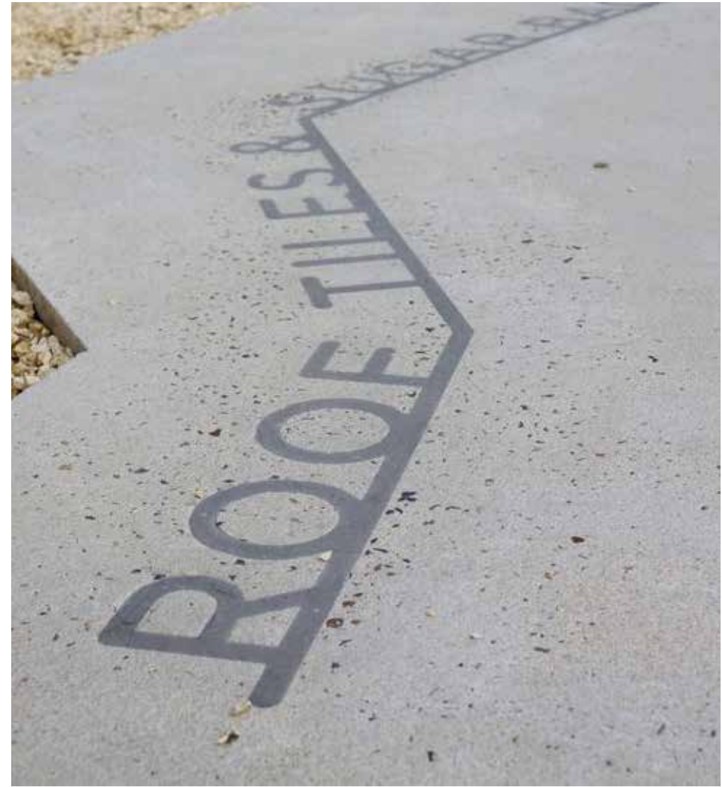
Laser cut text inlaid with insitu paving
