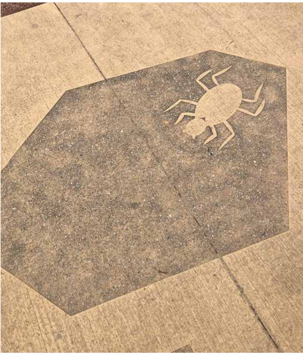
Design narrative: sand blasted concrete with stencil
