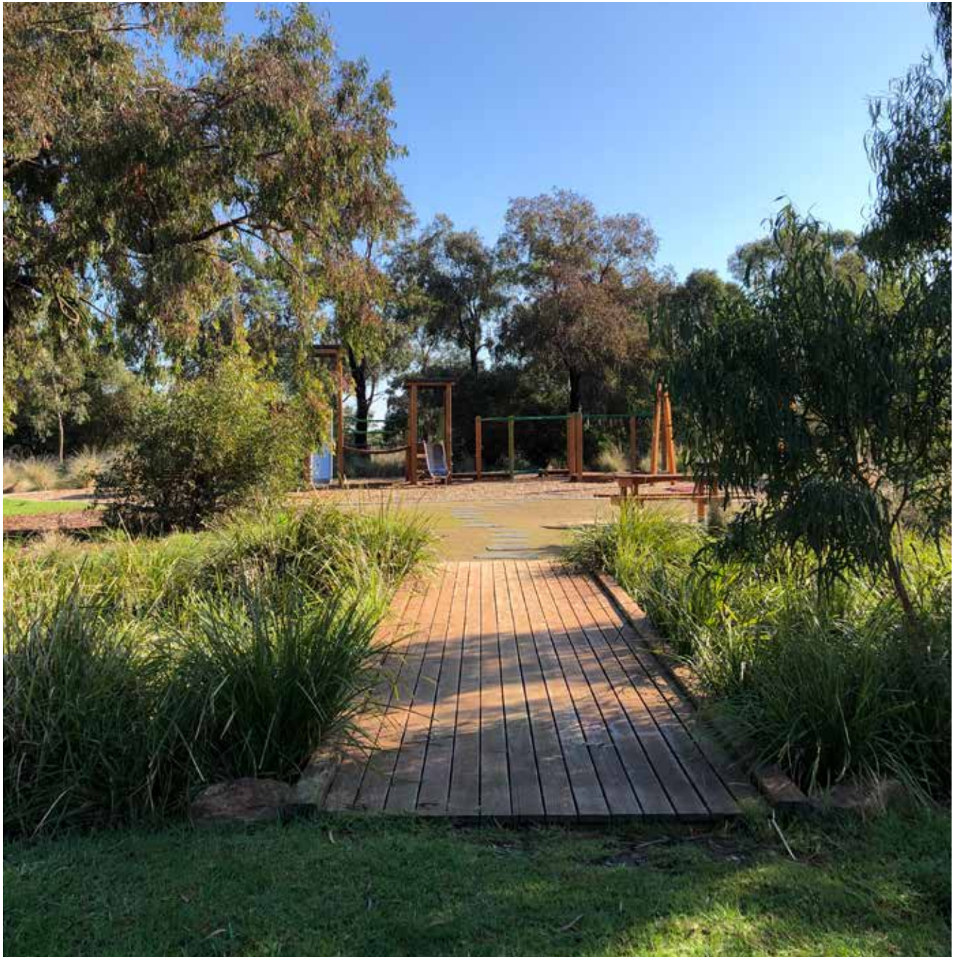
Existing timber bridge over swale does not connect to accessible sealed pathway
