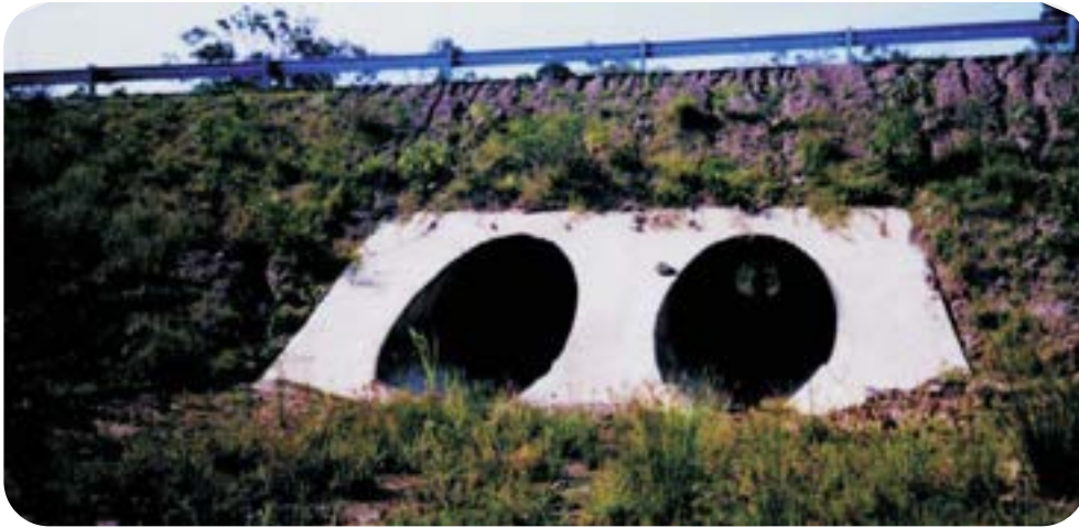
Image 15. A large culvert under a freeway providing passage for ground-dwelling fauna. Photograph from Queensland Department of Main Roads (2000).
