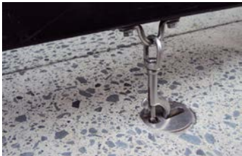
Figure 20: Acceptable Blind Anchor
