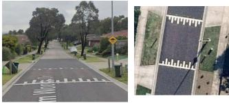
Raised slow points also add an additional benefit of narrowing the road width to allow one vehicle at a time. These treatments are only suitable for low traffic streets (less than 1,000 vehicles per day).
