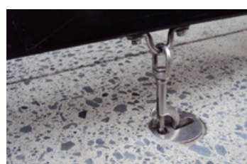
Figure 20: Acceptable Blind Anchor
