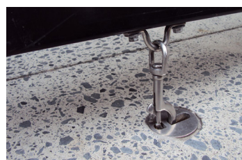
Figure 20: Acceptable Blind Anchor
